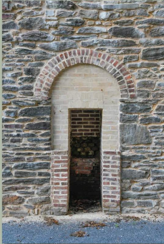
This northern-most kiln in the group is a continuous burn, vertical shaft kiln once owned by Thomas Risteau Jenifer. This 1883 kiln measures 14 feet square for its full 25 foot height. Its walls are at least 4 feet thick surrounding the circular center stack. The arched “poke holes” on either side were used to monitor the burning of the Cockeysville Marble and, when the time was right, to stoke or push the mass of marble and ash down to the cooling chamber below.
