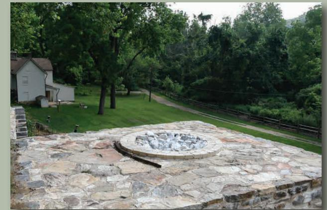
Atop the Jenifer Kiln stood a 10 foot to 15 foot high chimney which aided in creating an up-draft for hot air baking of the marble and in carrying away the smoke and toxic fumes from the lime making process. When the kiln was no longer in use, the chimney was collapsed into the kiln stack to prevent possible injury to people and prize dairy cows.
